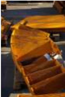
Lighthouse stairs awaiting restoration
