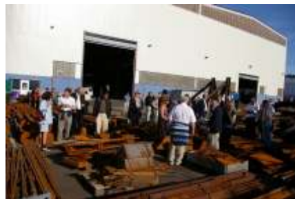
Parts of the Pater Noster Lighthouse after removal to Pharmadule Emtunga for restoration.
