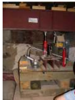
One of the jacks used to level the lighthouse.
