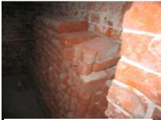
The remanufactured forming bricks.
