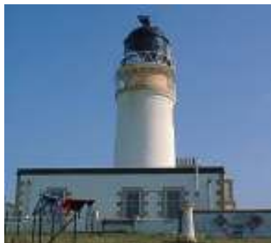
Killantringan Lighthouse Engineered by David Stevenson. First lit in 1900. Present characteristic flashing white (2) every 15 seconds. Candlepower 480,000. Nominal range 25 miles.
