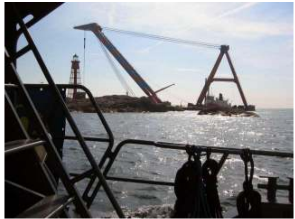
Pater Noster Lighthouse being lifted back onto its original home.
