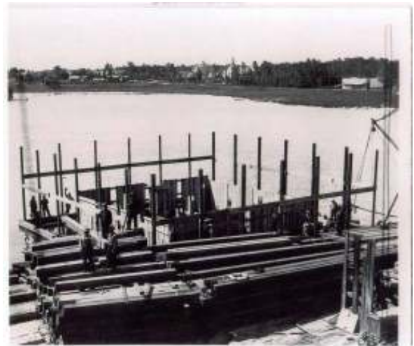
Original crib being built.
