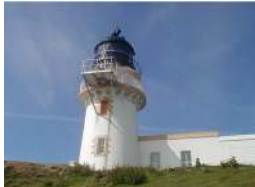
Tod Head Lighthouse Engineer was David Stevenson. First lit in 1897. Present characteristic flashing (4) white every 30 seconds. 3,000,000 candlepower. Nominal range 18 miles.
