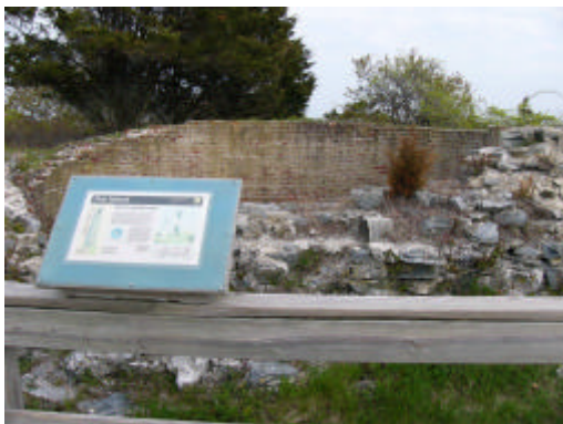
Ruins of the 1827 tower at Fire Island
