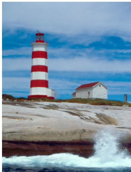
Sambro Lighthouse after restoration. The equipment building stands behind the lighthouse.
