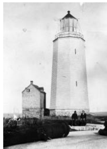
The lantern of 1864 and the accommodation for the Royal Artillery fog gun crew. A cannon lies in the left foreground, so we know this photograph was taken after 1876 when the fog gun was discontinued.
