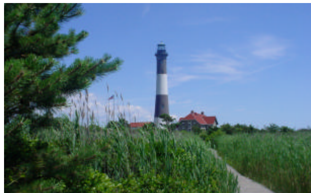
1858 Fire Island Lighthouse
