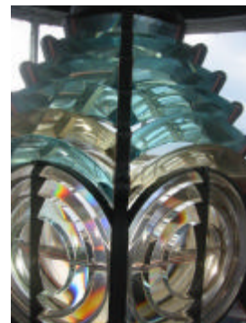
White prisms were originally made by Chance Bros., and blue prisms were made in Japan during the restoration.
